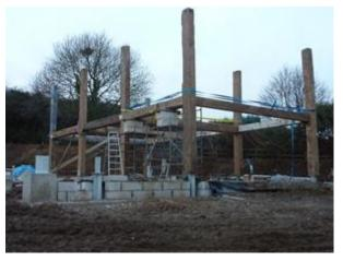
Lowen will be constructed using straw bales in a timber frame and lime rendered inside and out. It will produce power from photovoltaic panels on the roof, hot water from evacuated solar tubes and the house will be heated by a ground source heat pump drawing energy directly from the earth. Rainwater from the roof will be captured and used for toilet flushing. Its roof will be turfed
