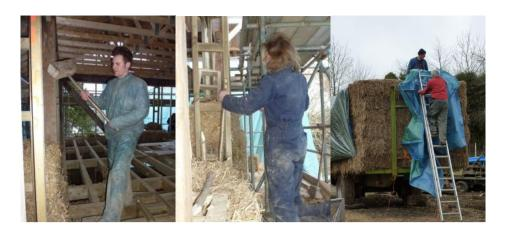
22/02/11 We've now got a specialist team from Natural Building Solutions working on the lime rendering. Straw needs good ventilation around it to stay healthy and the weatherproof material must also allow it to breathe so the ideal finishes are traditional lime or natural clay painted with limewash or breathable paint.
